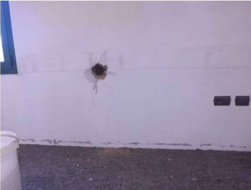
3) Detail of the pre-treatment work
