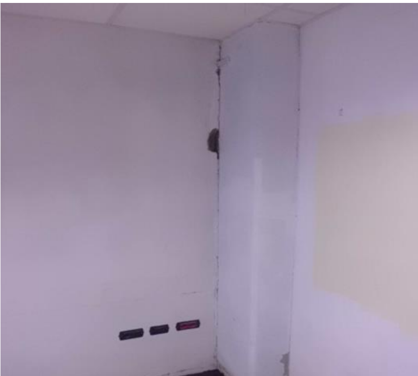
4) Detail of the pre-treatment work
